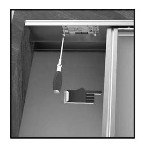
3. Open the door and screw the plate securely in place
